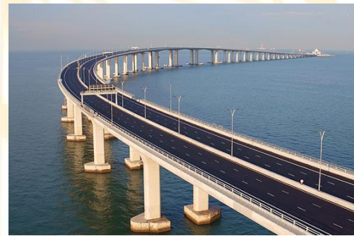
Hong Kong-Zhuhai-Macao Bridge
